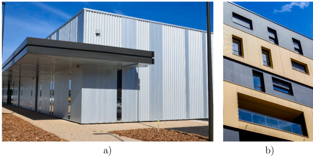
Fig. 2. Application of sinusoidal profiles: (a) SNC Pont d'Ouit (Architect: DGA-Architecture); (b) Aiguillon Construction (Architect: Christophe Roussele Architecte).
