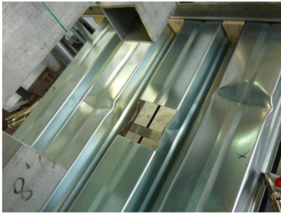
Figure B.7: Failure mode (exemplary for PF-4Hs1-075-1)
